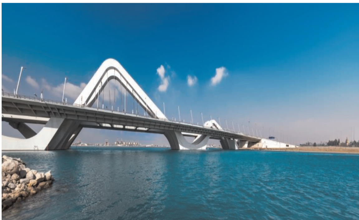
Figure 5. Sheik Zayed bridge [33].
