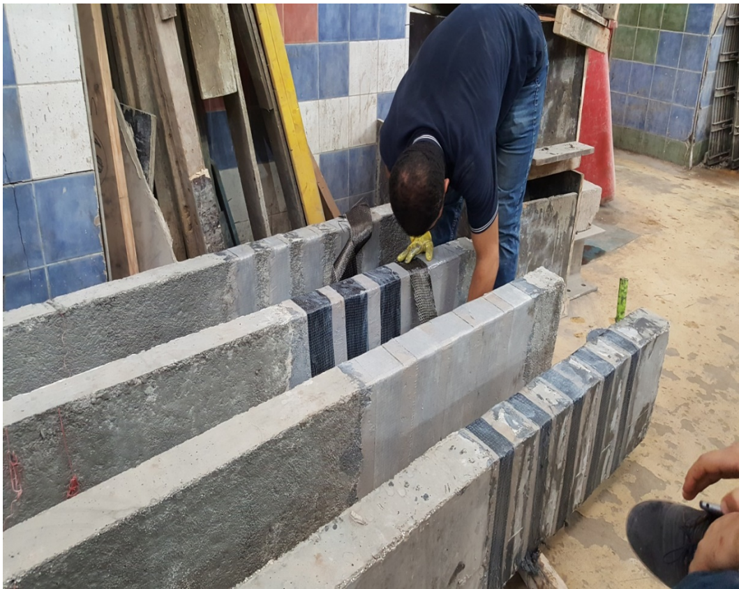
Figure 5 U-shape FRP wrapping
