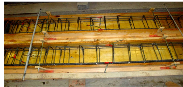
Fig. 3 Steel reinforcement of specimens in formwork.
