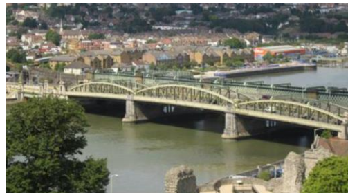
Fig. 1 – The Rochester Bridge, UK
