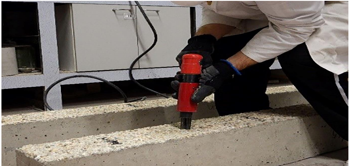
Figure 4 Roughening of the surface with a pistol grip needle scaler
