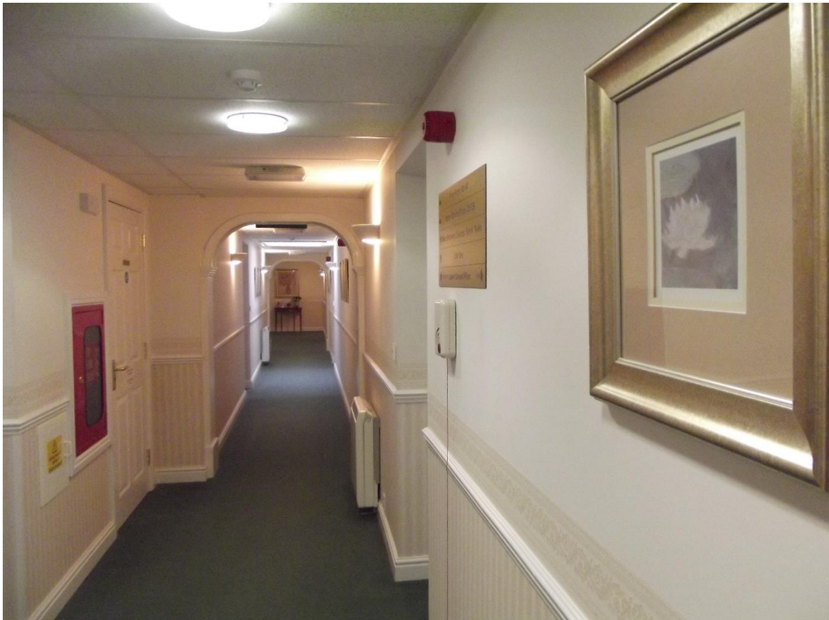
Figure 2: Image of communal corridors.
