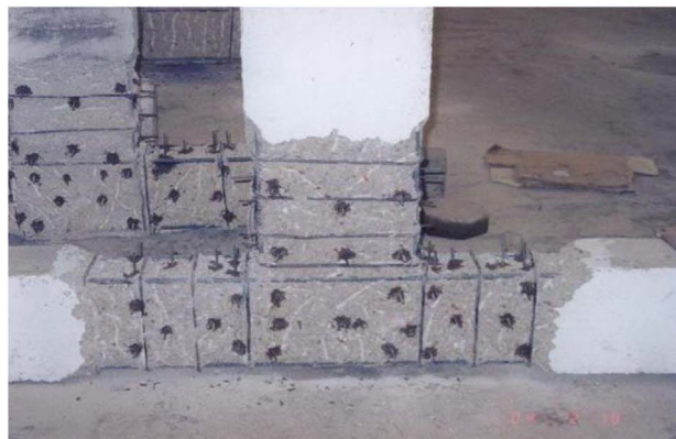
(b) Drilling holes and inserting steel dowels
