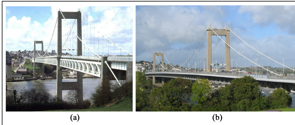
Figure 2. Tamar suspension bridge (a) before (1978) 36 and (b) after (2018) its reconstruction in the late 1990s. Note the larger deck and stay cables added in 2001.
