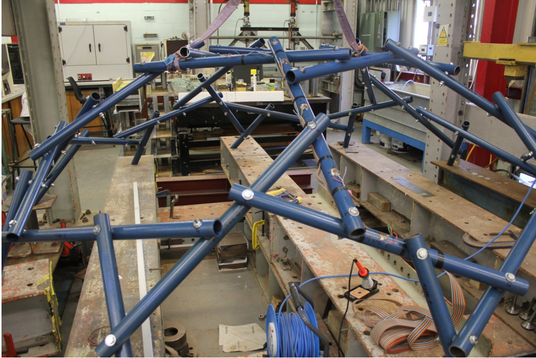
Figure 7: Honeycomb dome being constructed in the laboratory.
