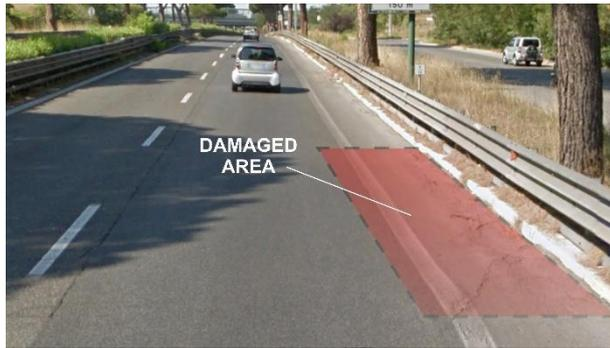
Fig. 1 – An example of asphalt damage due to the uplift of tree roots at the edge of the lateral lane and at the verge
