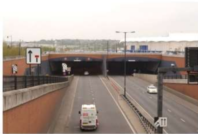
Fig. 2. Medway Tunnel eastbound entrance.
