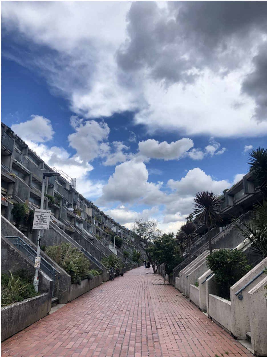
FIGURE 5 Rowley Way, Alexandra Road Estate.
