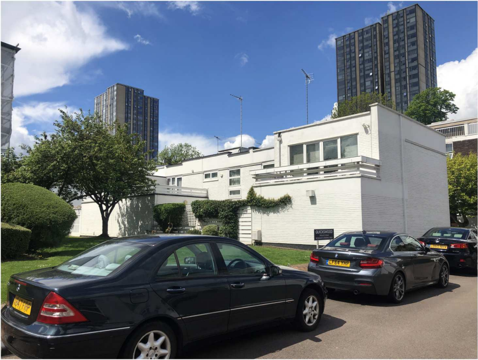
FIGURE 3 High-rise and low-rise housing on the Chalcots Estate.
