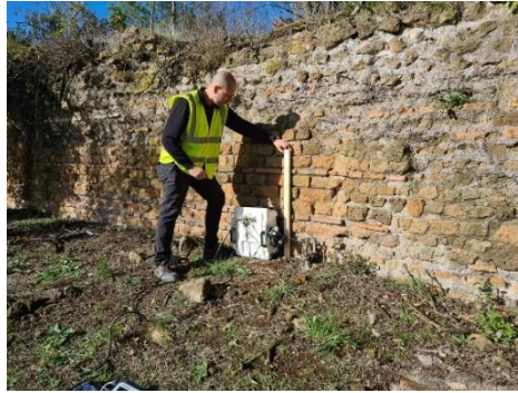
Fig. 3. GPR data collection on the perimeter stone masonry wall at the Circus of Maxentius.
