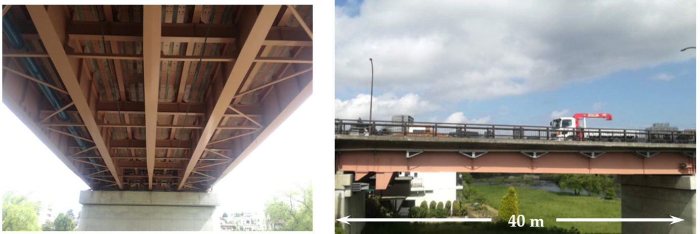
Figure 20. Concrete road bridge under measurement.
