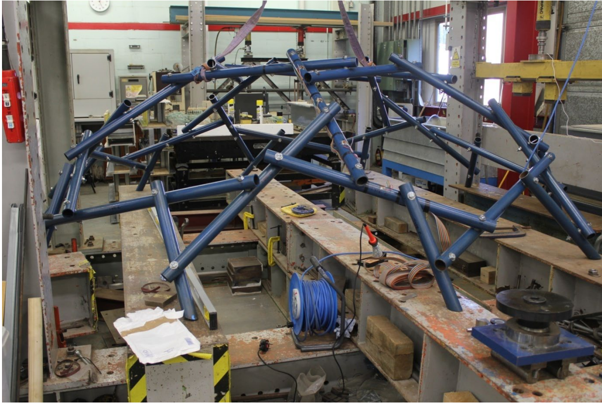
RSE honeycomb dome being constructed.
