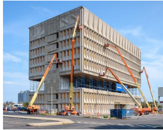
Figure 19. The building under refurbishment (Stouhi 2021)
