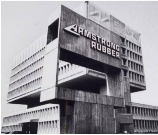
Figure 18. Pirelli Tire Building original form (Forre n.d.)
