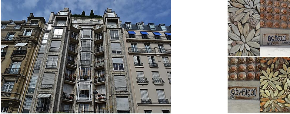
Figure 3. Perret's Rue Franklin reinforced concrete building clad with terracotta tiles (Invisible Paris 2013)
