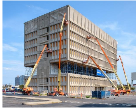
Figure 19. The building under refurbishment (Stouhi 2021)
