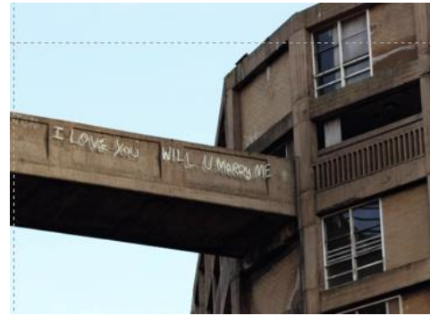
Figure 13. Park Hill Estate, Sheffield – Roads in the sky (Moustaka 2023)
