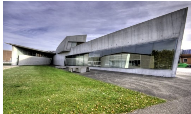
Figure 13 Vitra Fire Station – Zaha Hadid 1993
