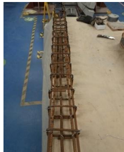
(b) Reinforcement cage for mild steel reinforcing bar
