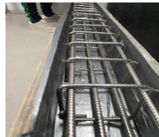
(f) Reinforcement cage for control stainless steel beam
