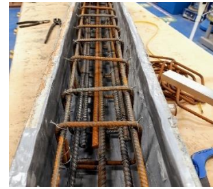
(c) Reinforcement cage with lap bars
