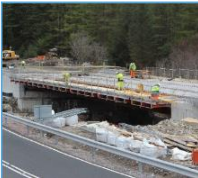
Figure 2.18. Allt Chonoglias Bridge in Scotland (Stainlessrebar, 2021)
