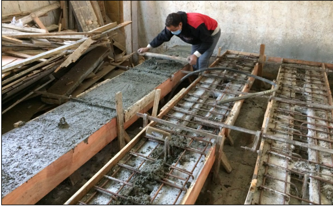
Figure 14: Casting concrete for the rest of topping slab (G2 to G6)
