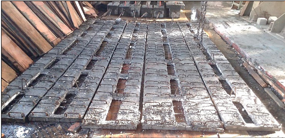
Figure 11: Lower part of topping slab (precast)
