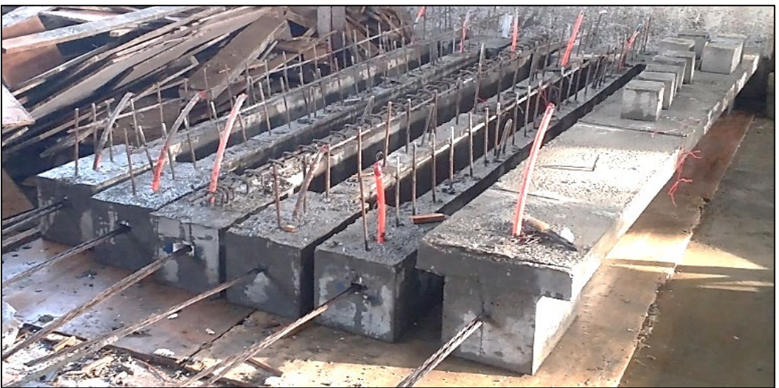
Figure 10: Control specimen G1 and five girder webs
