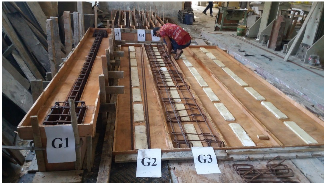
Figure 8: Preparation of reinforcement for tested specimens
