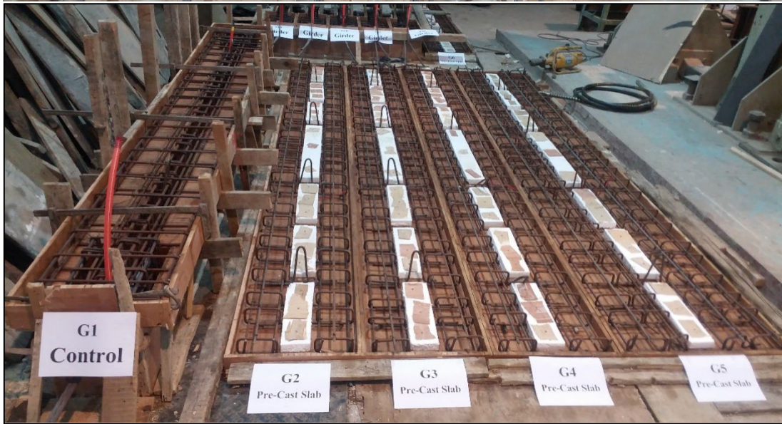
Figure 9: Finishing preparation of reinforcement for all specimens
