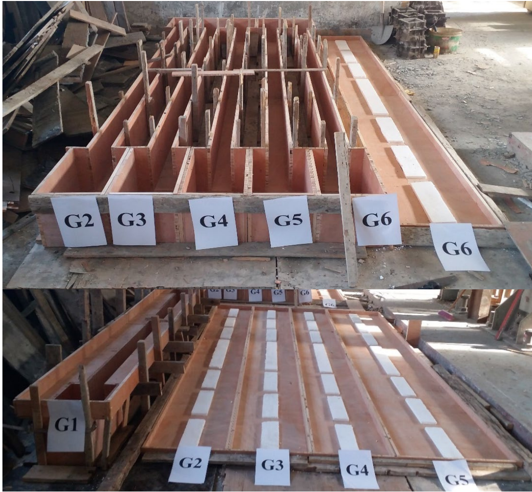
Figure 7: Preparation of formwork for tested specimens
