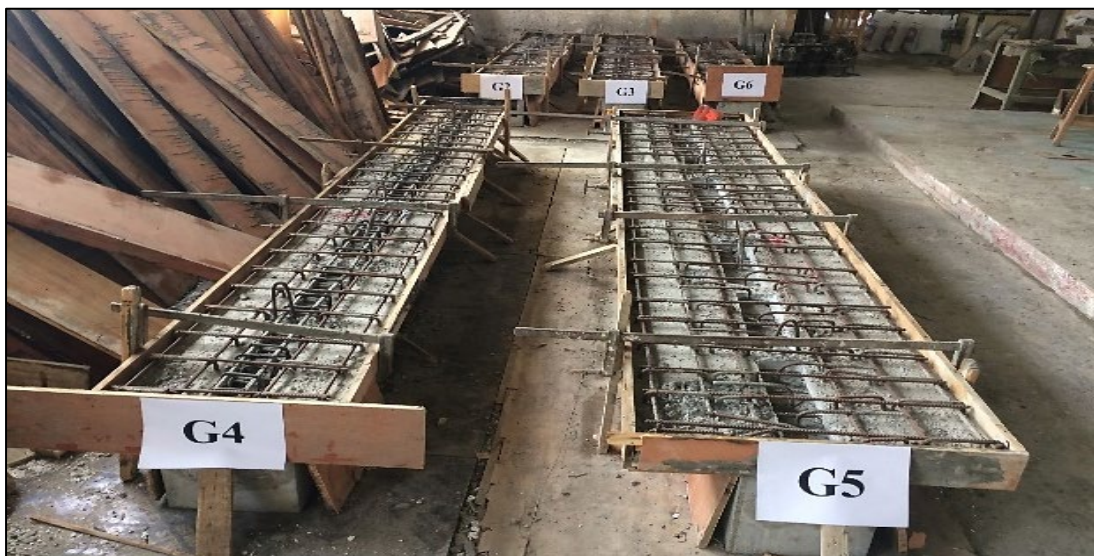
Figure 13: Preparation of casting the rest of topping slab
