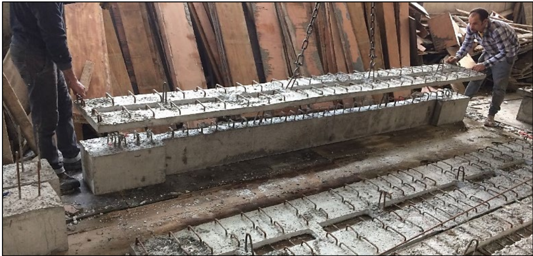
Figure 12: Installation of the lower part of topping slab above girder web
