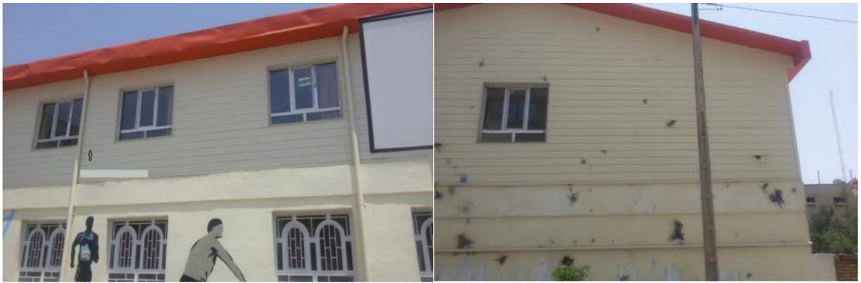
Figure 22. Dry facades problems in LSF system: right panel: striking some heavy things to dry facades. Left panel: bad performance of construction or insulation
