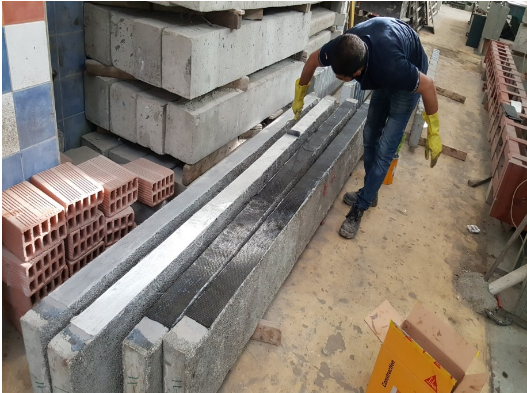
Figure 4 Attaching the FRP layers on bottom surface of studied beams
