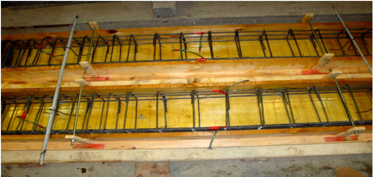
Figure 3 Steel reinforcement of specimens in formwork
