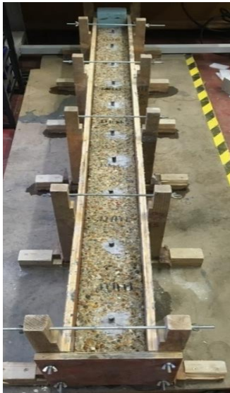
Figure 3 Beam with dowels ready for casting
