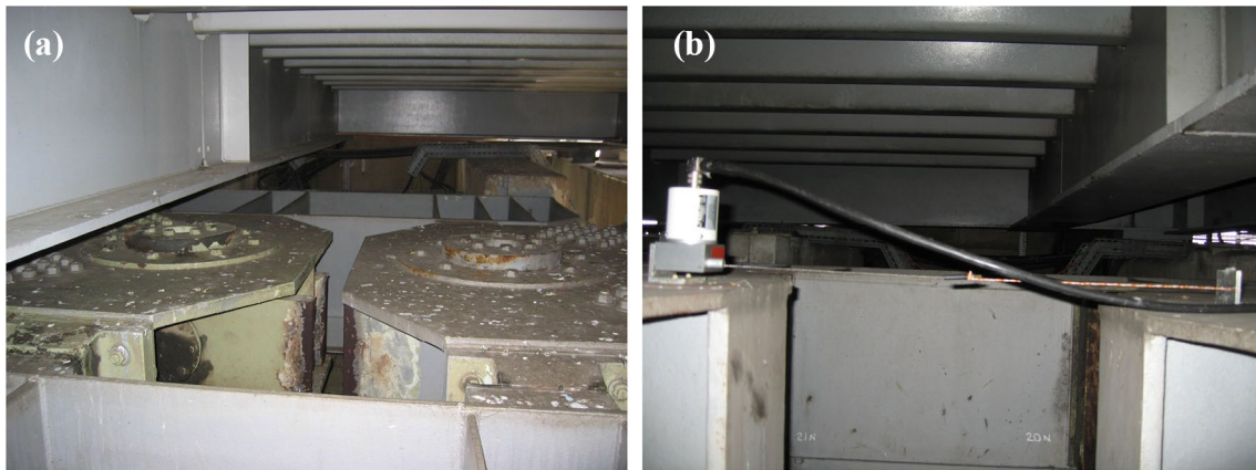
Fig. 5 New bearings at the Saltash tower (a) and setup of string gauge for measurement of the expansion joint thermal dilation (b)
