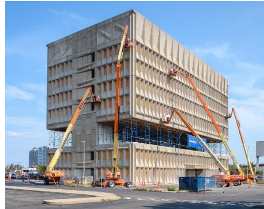
Figure 19. The building under refurbishment (Stouhi 2021)
