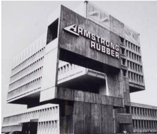
Figure 18. Pirelli Tire Building original form (Forre n.d.)
