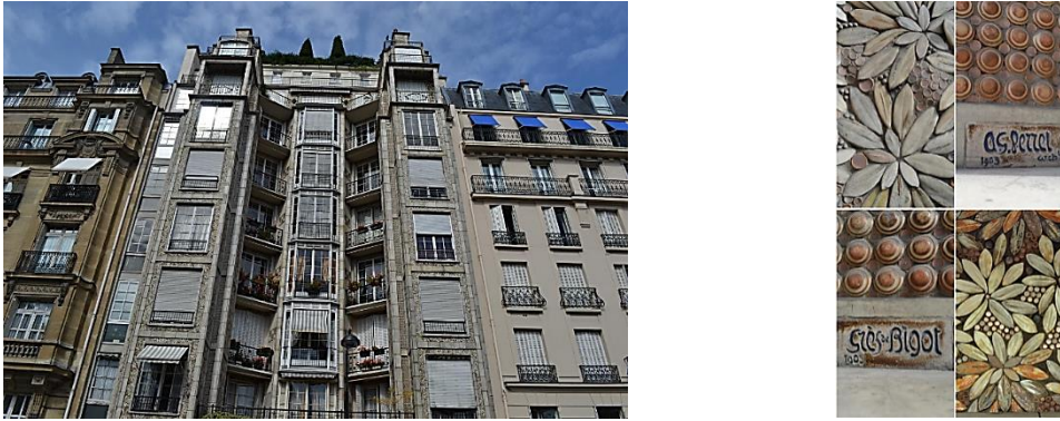
Figure 3. Perret's Rue Franklin reinforced concrete building clad with terracotta tiles (Invisible Paris 2013)
