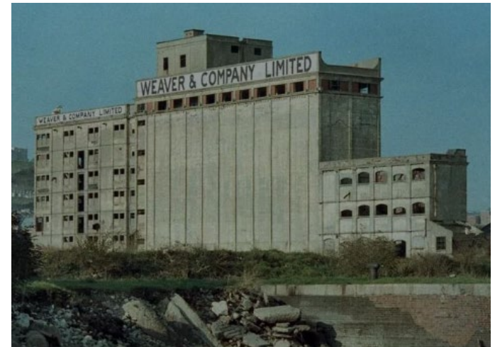
Figure 2: Hennebique building in England; Weaver Company 1898 (Historic England 2022)
