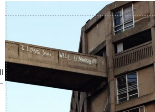
Figure 11 Park Hill Estate, Sheffield – Roads in the sky (Moustaka 2023)
