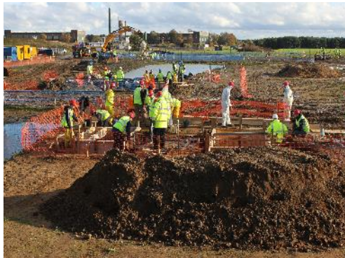
Foundation shuttering being installed after being set out
