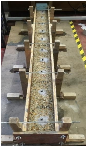
Figure 3 Beam with dowels ready for casting
