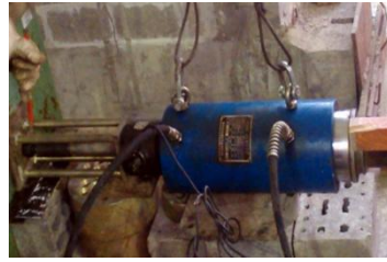
b) Prestressing the CFRP rods.
