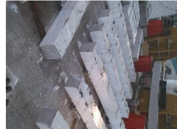
f) Strengthened beams.
