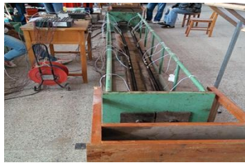
a) Installation of CFRP rods.
