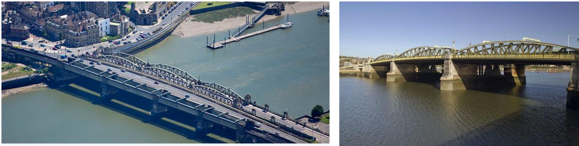
Fig. 1. Main features of the Rochester Bridge, UK
