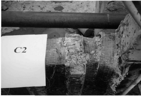
Figure 10 Failure of Specimen C2
