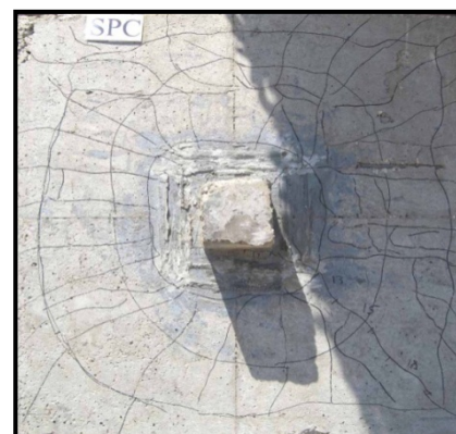
Cracking pattern of specimen SPC
