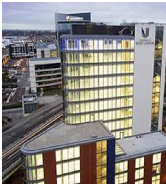
Figure 7 View of the Paragon building (Source uwl.ac.uk )
