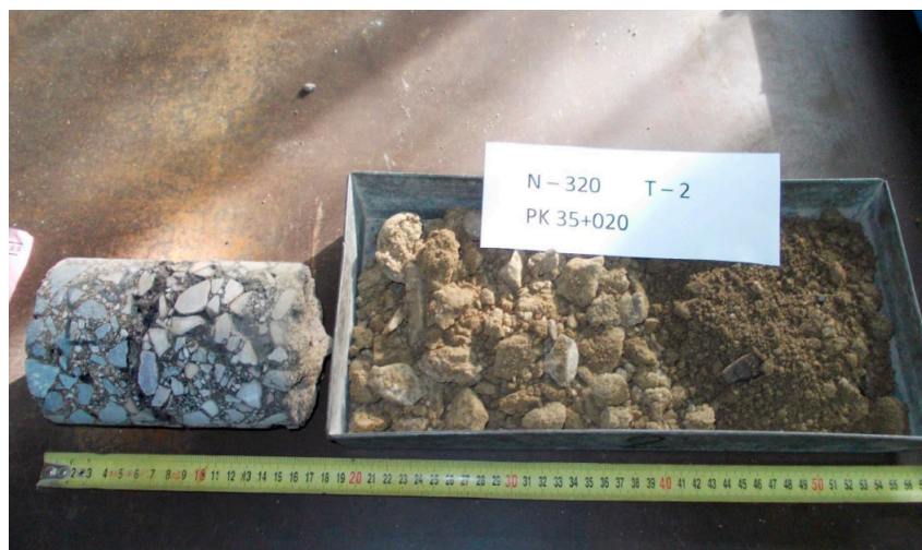
Figure 4. Pavement structure by a reference sampling core.
