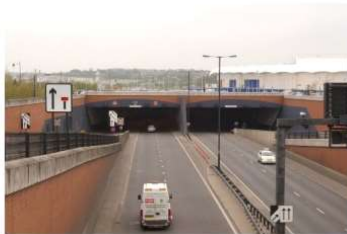
Fig. 2. Medway Tunnel eastbound entrance.
